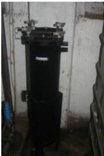
**Figure 18** Stainless steel filter housing unit for a bag filter (without pump or storage), at Diligent Tanzania Ltd.
